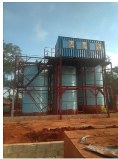
CIP Tanks and Control Room
